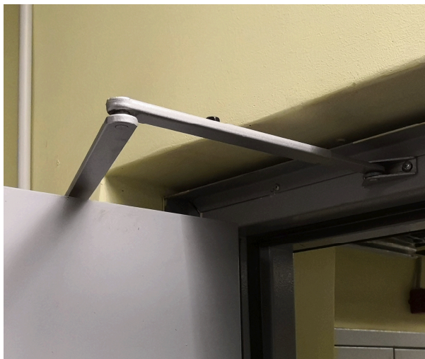
Pašaizveres mehānisms, kas aizvēra durvis Magnēts, kas tur durvis atvērta stāvokli Self-closing mechanism that closed the door A magnet that holds the door in the open position
